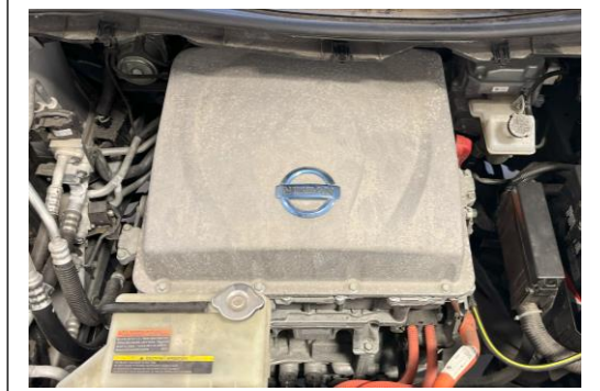
Removing the lid with the Nissan logo will expose the electronics for the DC-DC converter and the HV AC and DC charger.
