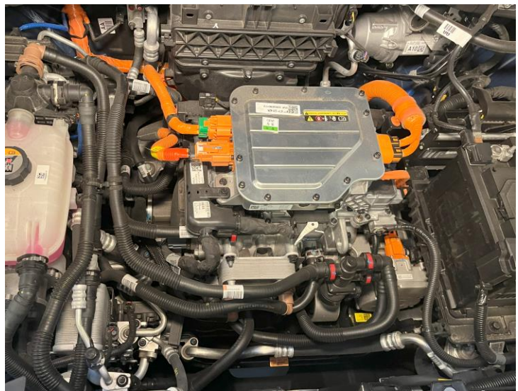
Under the hood of a KIA EV 6, the box on top is the front motor inverter with battery power entering the right side, AC compressor power leaving the lower right, and PTC heater circuits leaving the left side.
